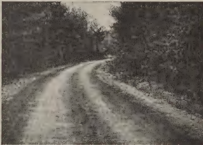
Oiled Road Not Rutted Because Travel Spread Around The Corner
